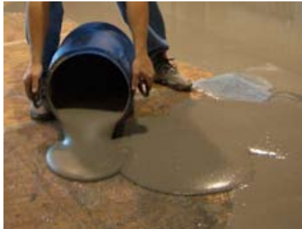
Self leveling underlaments (SLUs) are an option in achieving a flat substrate. Photo courtesy of ProSpec.
