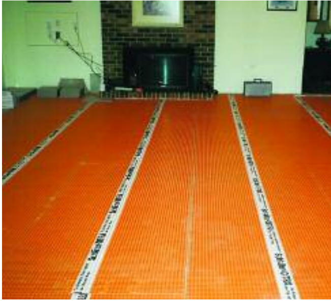
Left: Some membrane systems allow for use as an underlayment in addition to offering crack suppression or waterproofing values. These added features plus the problem solving reduced height profile are all rolled up into one product.
